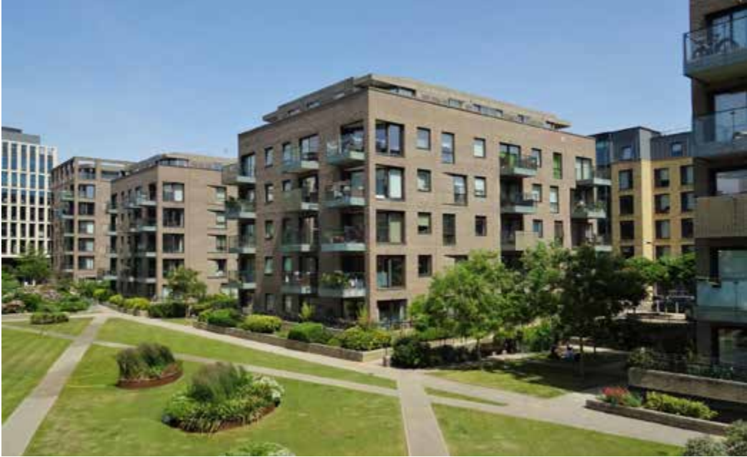
Mill Park refurbishment scheme, Cambridge
