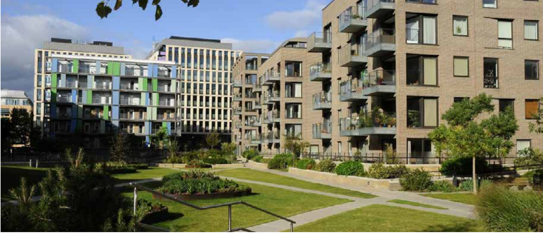
Mill Park refurbishment scheme, Cambridge
