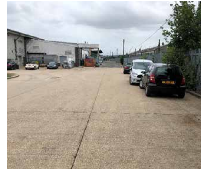
Existing site looking north adjacent to railway
