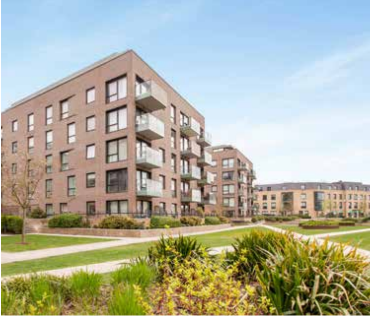
Mill Park refurbishment scheme, Cambridge
